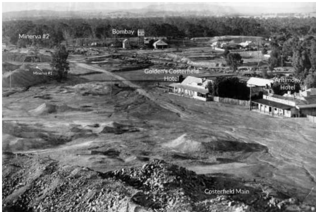
Figure 6. Costerfield ca. 1914, photograph taken from the Costerfield Main headframe looking south-east.
